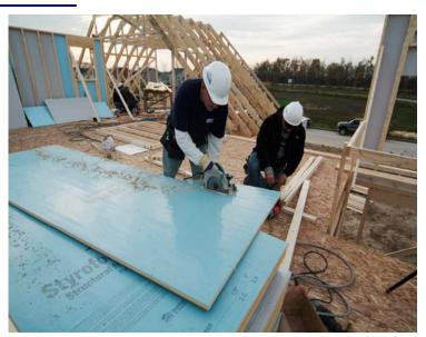
structural bracing and water-resistive barrier. When used as structural bracing, STYROFOAM SIS can be installed continuously, or intermittently with another insulating sheathing. Both options meet the requirements for "continuous insulation," a building practice that is quickly gaining favor among regulators and industry rating systems for its ability to significantly increase energy savings by addressing thermal shorts and preventing air infiltration.
